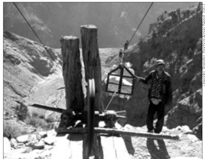
Gravity Ropeways in Nepal, an environmentally and economically viable alternative to roads in mountainous areas.
